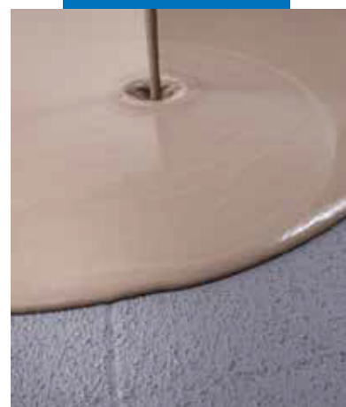
Application of self-levelling smoothing compound on dry Eco Prim Grip Plus on old floor
